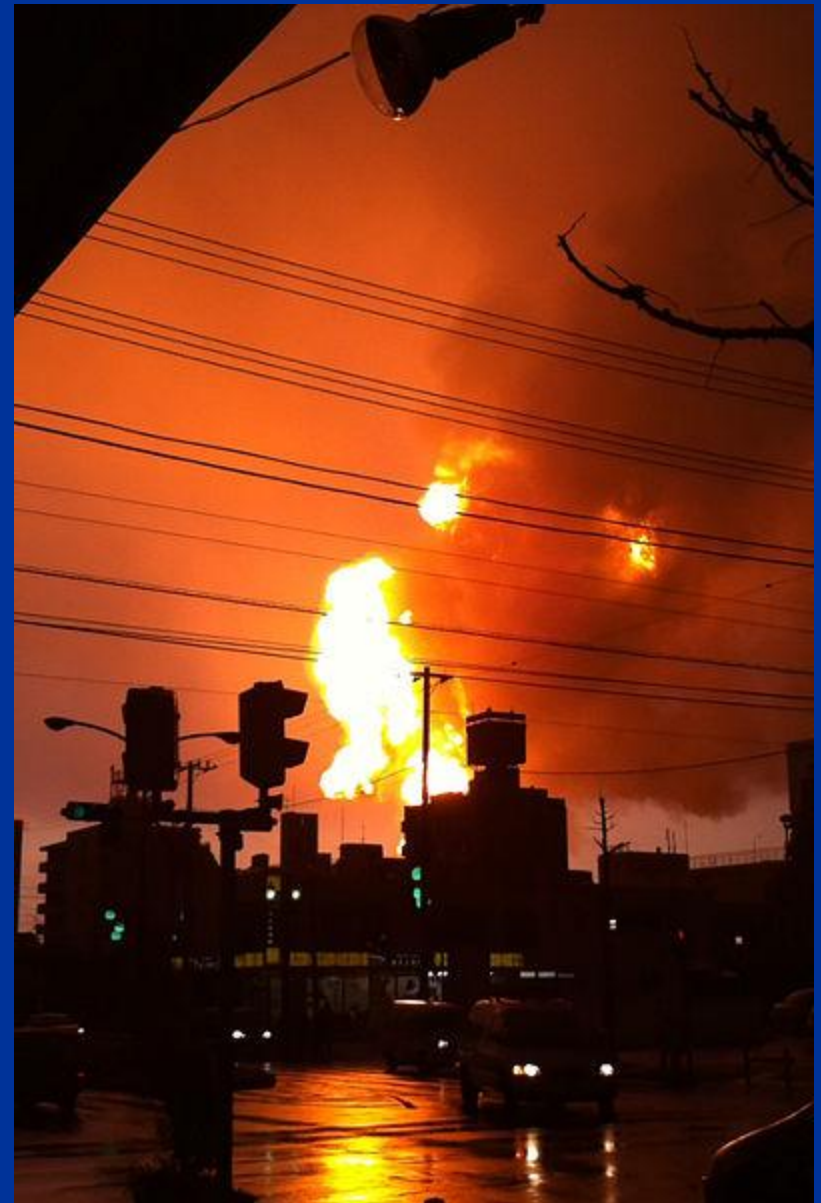
Fire at the Cosmo Oil refinery in Ichihara
