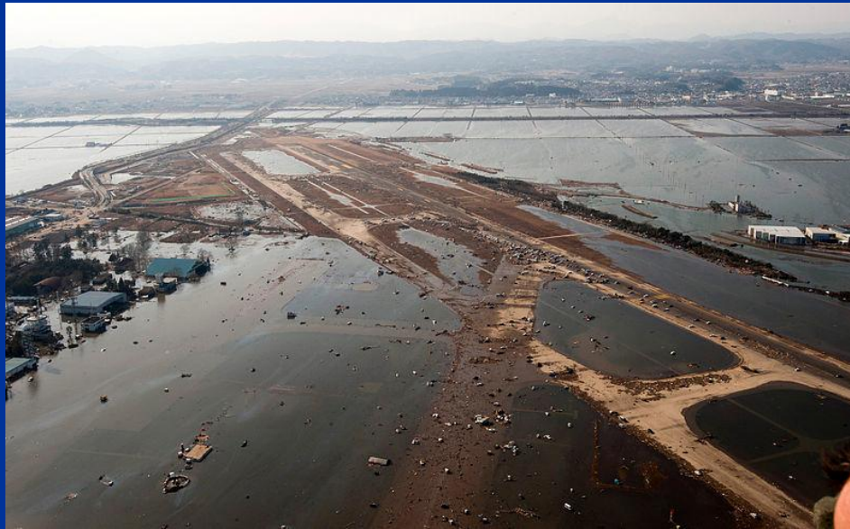
Tsunami flooding at Sendai airport
