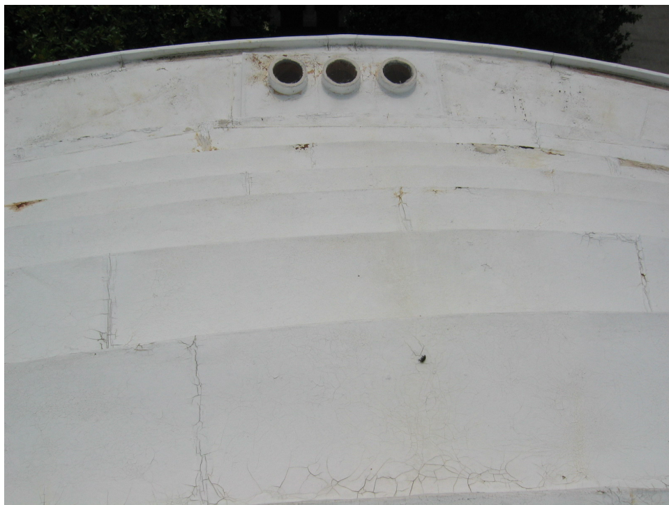
The skylight (top) and the west chimney (bottom). [JGWA, 2006]
