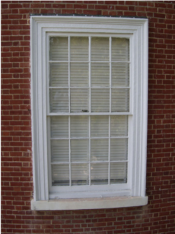
East elevation Dome Room window. ([JGWA, 2006]
