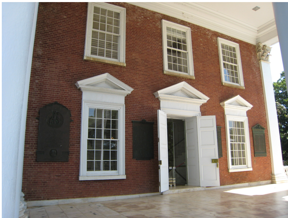
South portico ceiling (top); south elevation (bottom). [JGWA, 2007]
