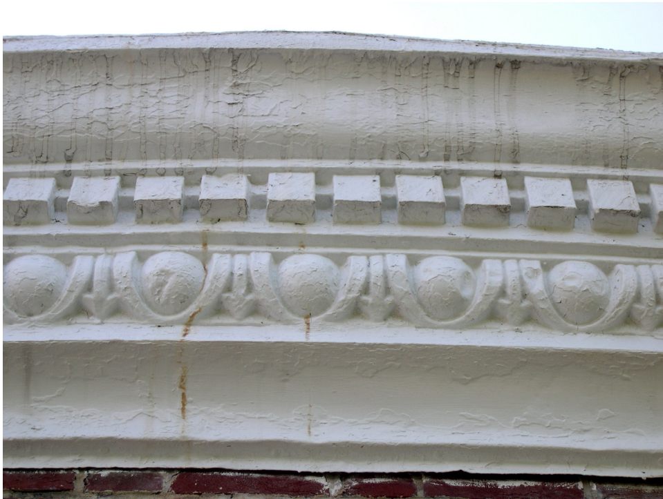
The cornice gutter and the base of the attic story (top); the crown molding at the top of the attic story (bottom). [JGWA, 2006]
