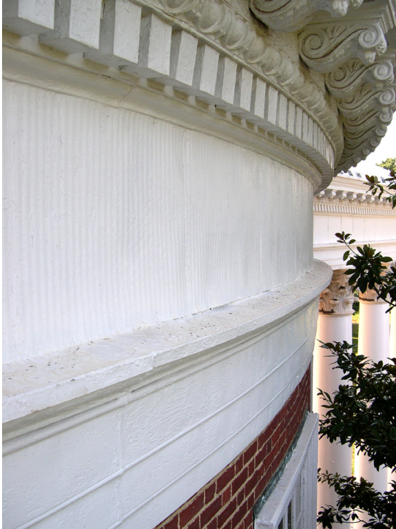
The entablature architrave and frieze (left), and cornice (upper left). [JGWA, 2006]
