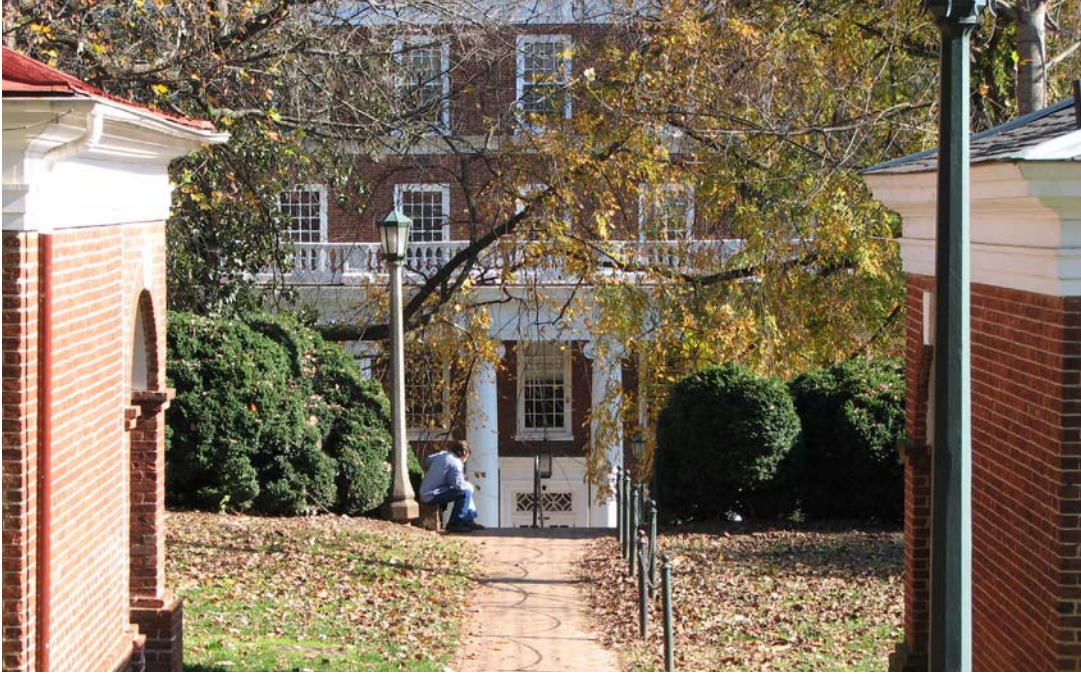
D: Existing connection between the Lawn and the West Complex
