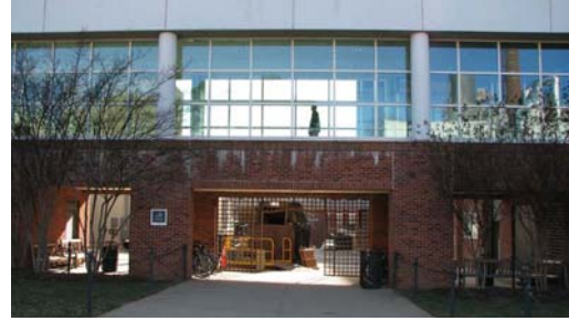
D1: Looking south toward the link and Jordan Hall/Primary Care Center alley
