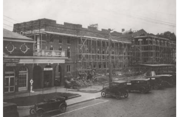
Medical School portico under construction, ca. 1928
