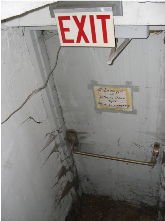
The emergency exit door (left) and floor slab (above) of the Northwest Fire Stair (C117) are dirty and covered with cob webs. The illuminated exit sign is not working. [JGWA, 2006]
