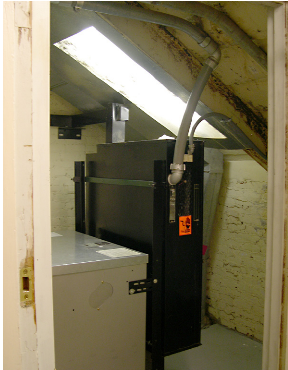
Elevator Machine Room (110A) below the North Portico. [JGWA, 2006]
