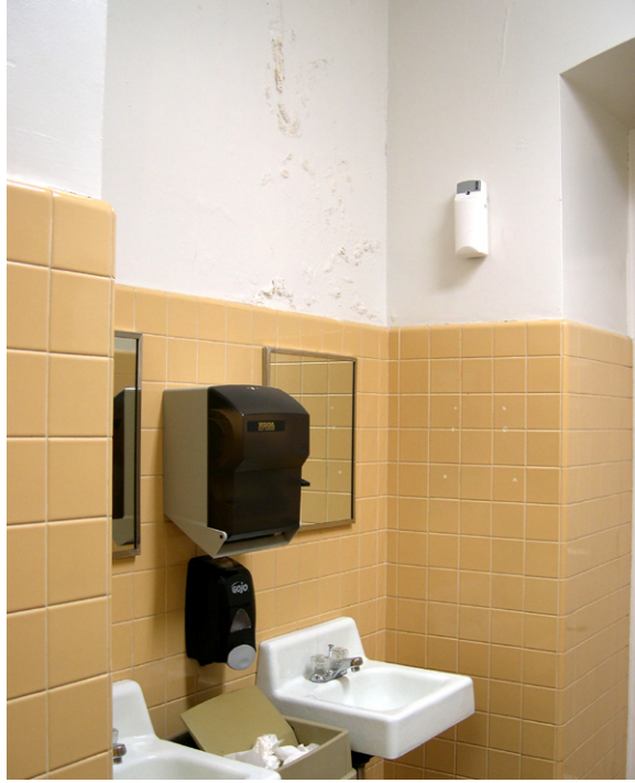
Men's Toilet Room (T113), looking northeast. [JGWA, 2006]
