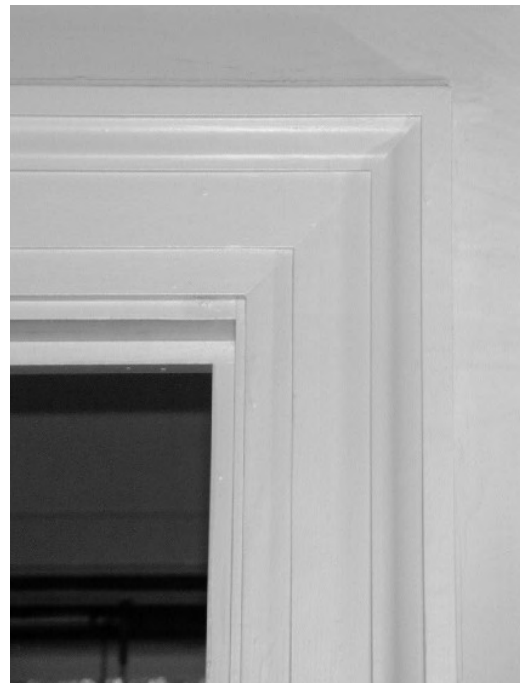
The doorway opening at the main first-story room has traditional mitered casings and backbands (right).
