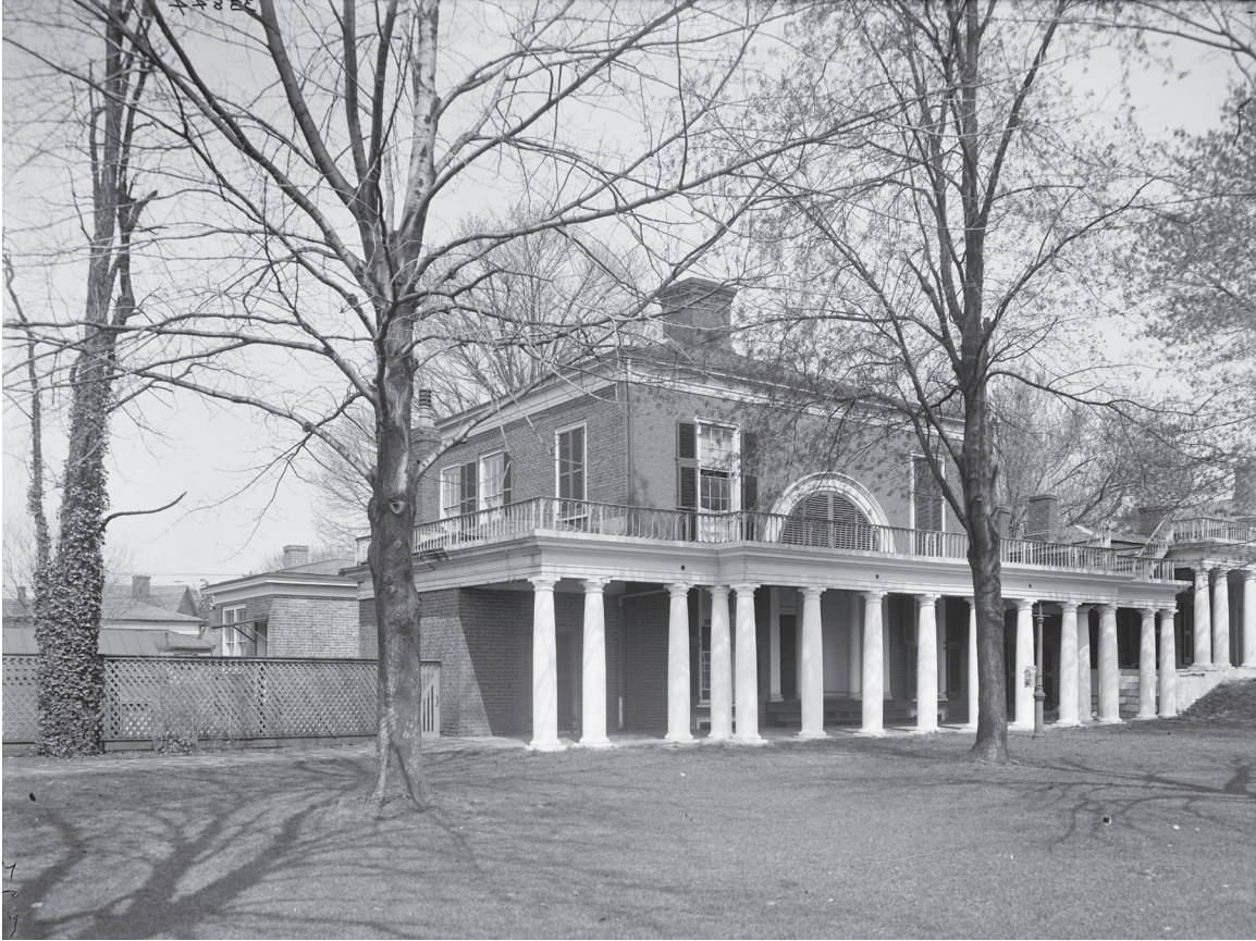
Pavilion IX, circa 1900-1910, by the Detroit Publishing Company; note the southwest addition with the doorway in the south elevation, and the shutters in the arch of the recessed entrance niche
