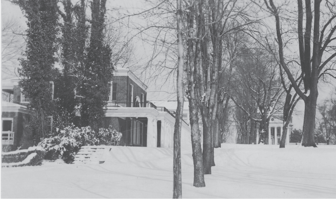
Pavilion IX from the south, 1900, showing the southwest addition
