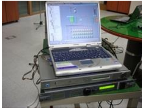
Figure 9. DSP equipment and howling detector.
