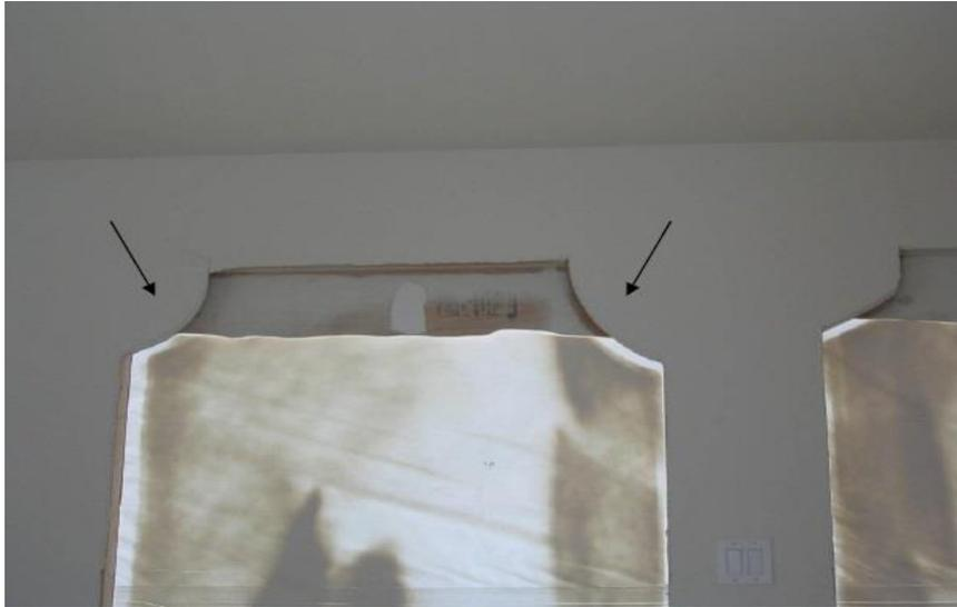
**Figure 18. Sheetrock is Cut with Extra Slack**
