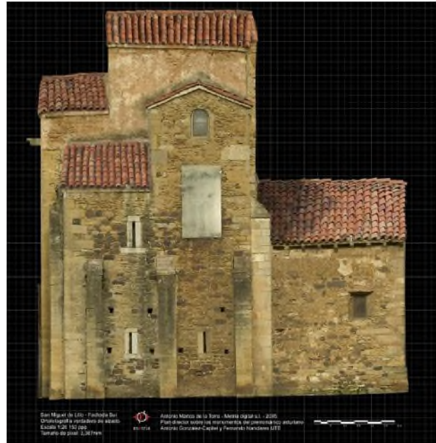
Figure 9. Final scaled orthoimage, composed from 9 different façade portions that match precisely
