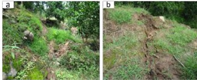
Fig. 3 Photographs of the ground cracks in the middle part of the eastern landslide in July 2007.
